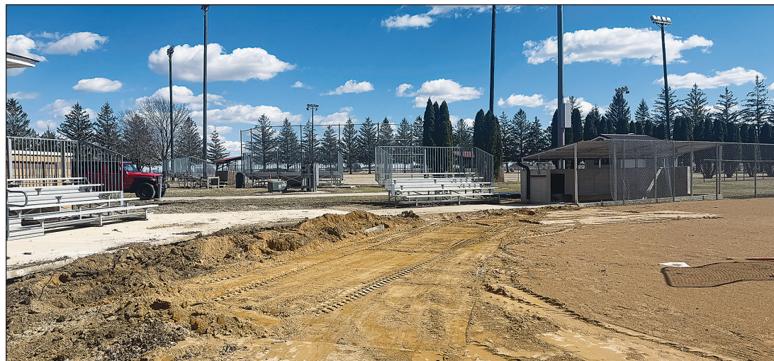
Work has started on a major renovation to the New Hampton High School varsity softball diamond at Mikkelson Park.
