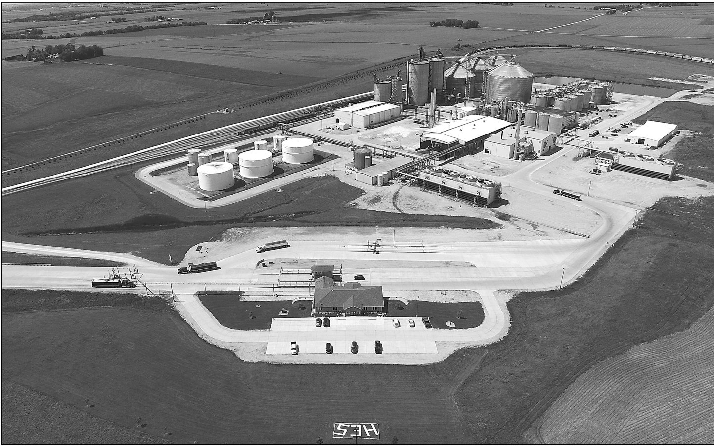
Photo courtesy of Homeland Energy Solutions
