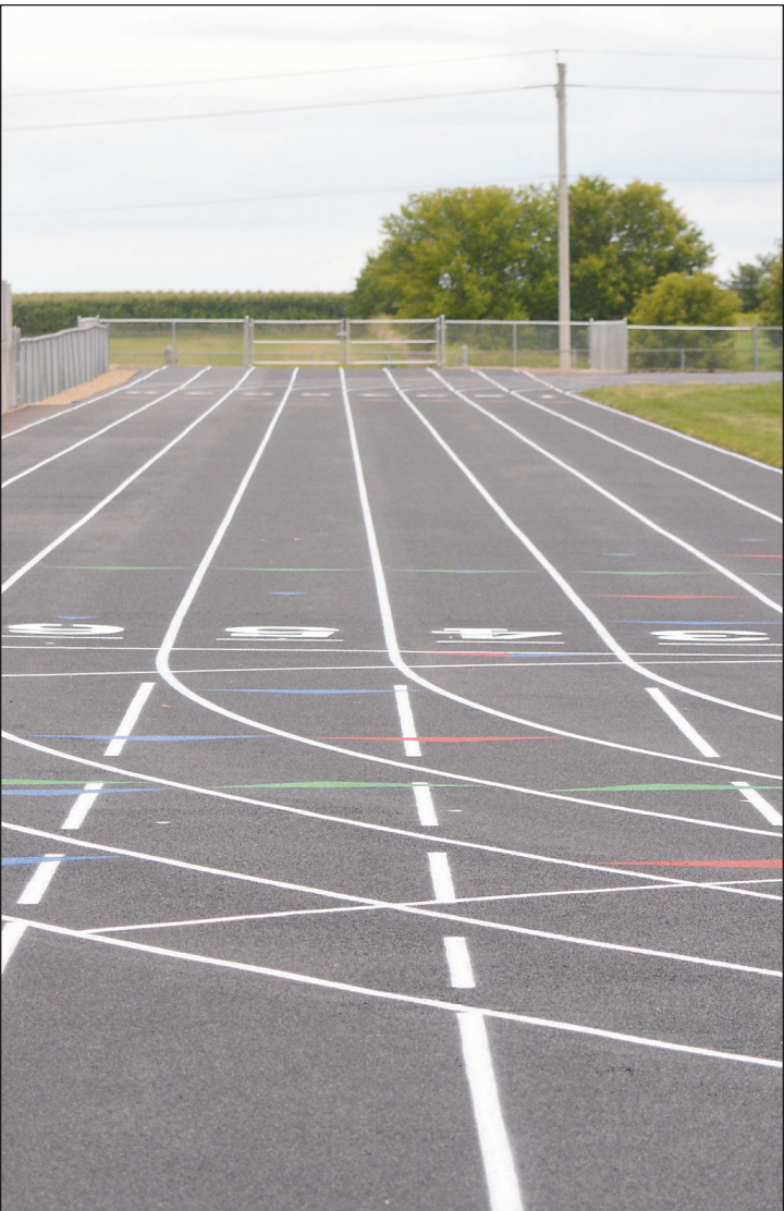
Bob Fenske/Tribune Work, including the painting of lines, on New Hampton High School’s new track was completed earlier this month.
