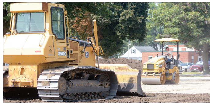
Bob Fenske/Tribune Ray Bachman spends Tuesday morning grading what will soon be the Kindness Square inclusive park at Runion Park.
