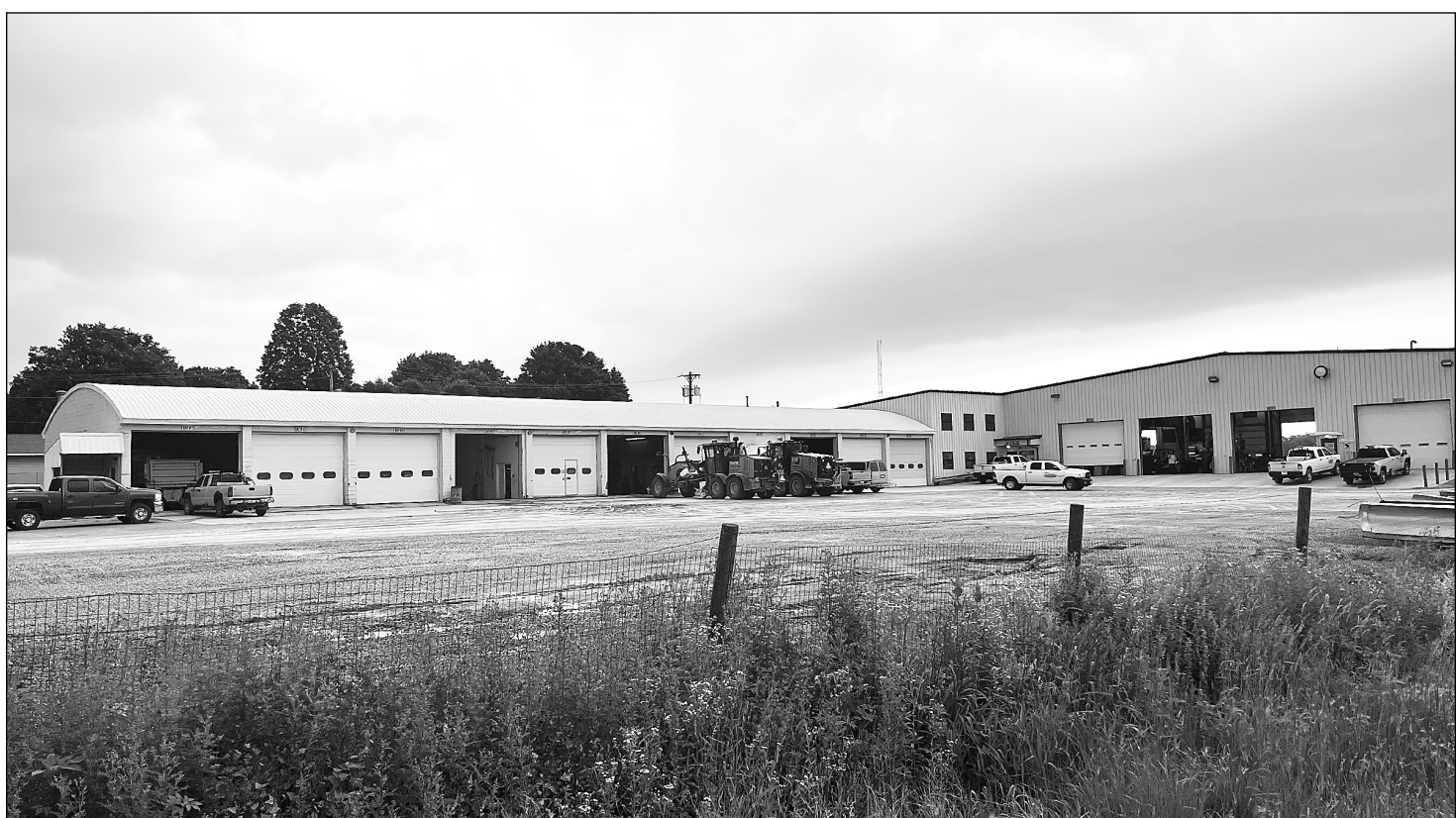
The Secondary Roads Shop that is located at 1990 Mission Ave. in New Hampton could be home to the County Engineer's Office.
